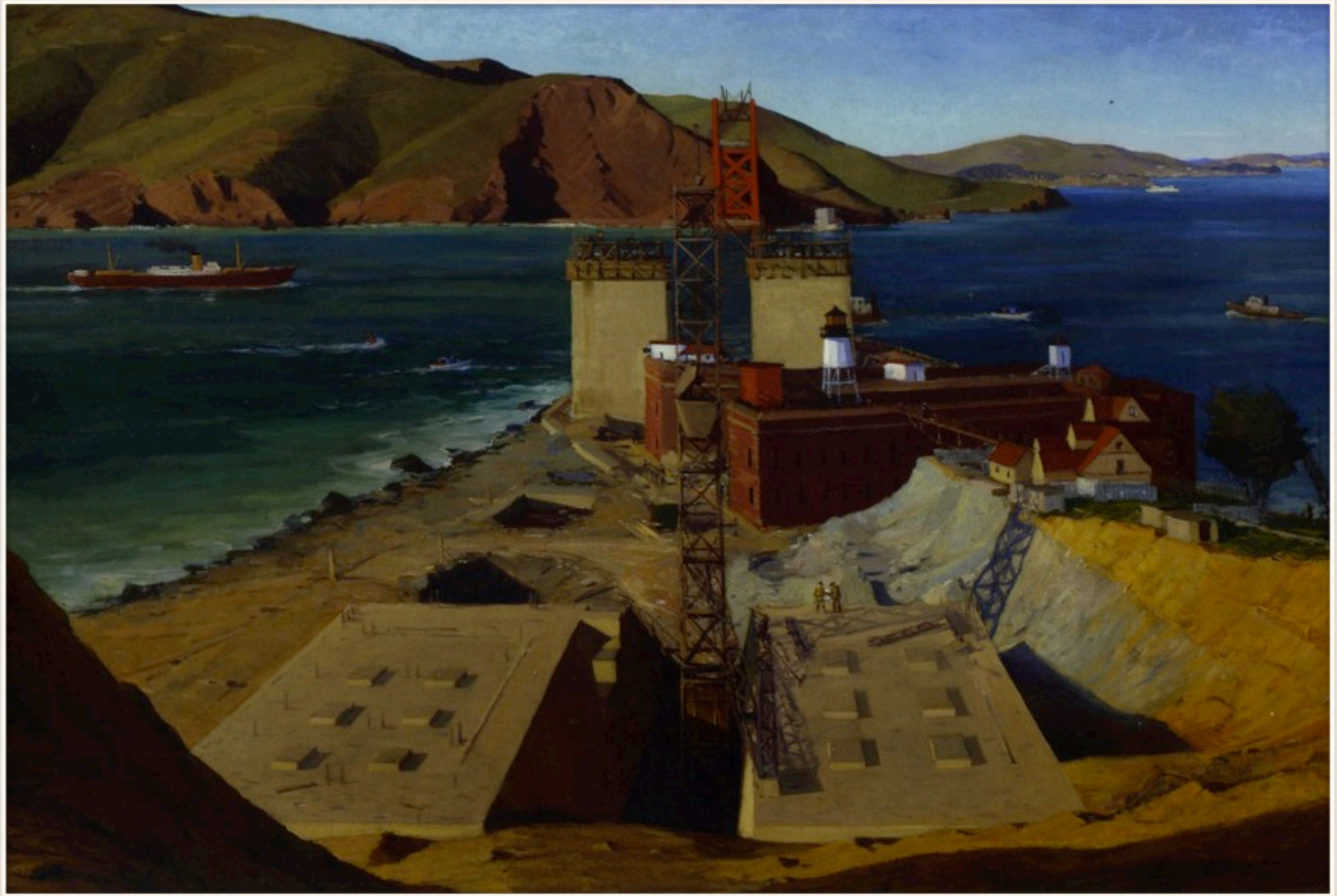
RAY STRONG, Golden Gate Bridge Under Construction , 1934
