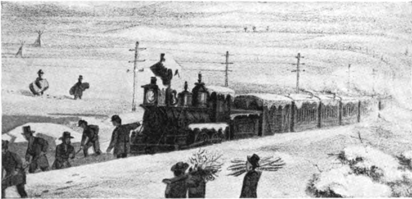
396.—An occasional experience of travellers on the first Pacific railroad after it was finished. They still had to get out and help, in one way or another, as they had done in the days of the keel-boat, Flying Machine and stage-coach.
