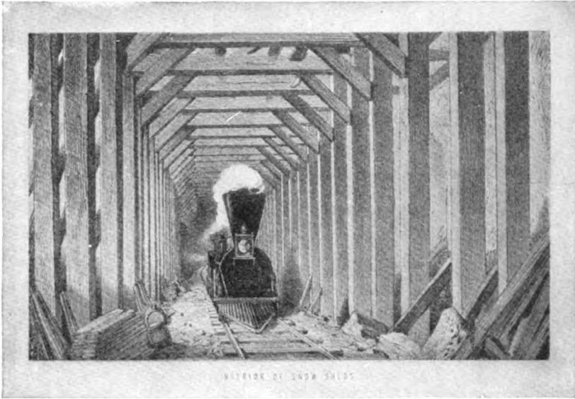
397.—Method of protecting trains from avalanches in the Sierra Nevada Mountains. Many miles of snow sheds had to be built.
